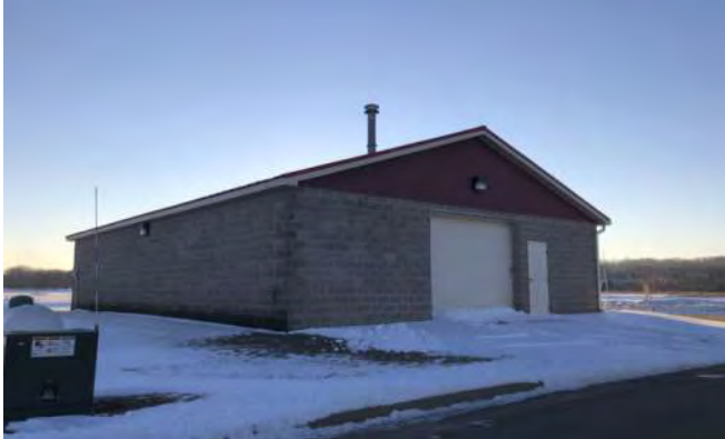
Rochester Youth Football Storage Building
