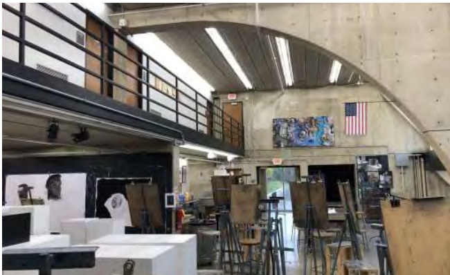
Upper Level Walkway
