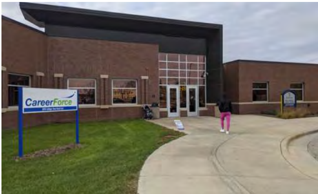
Heintz Center Main Entry and Drop-off Area
