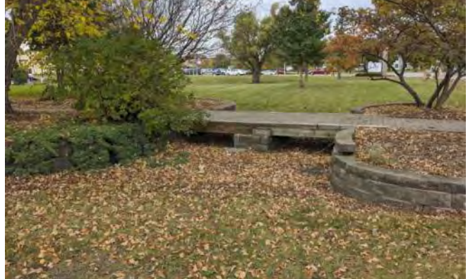
Pedestrian "Bridge"- Student Project North of Heintz Center
