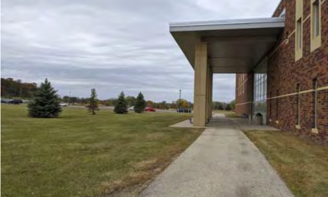
Small Gathering Area Near Sports Center South Entry
