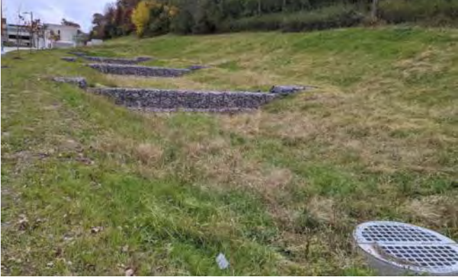
Stormwater BMP Near South Courtyard and Woods
