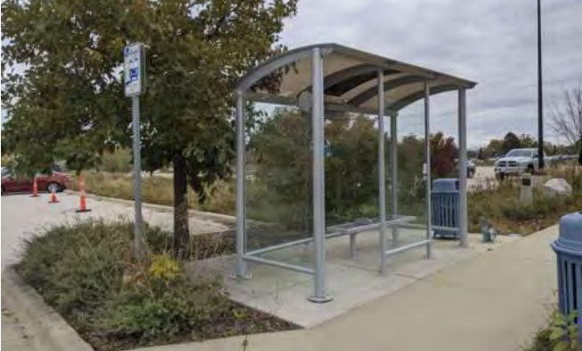
Park and Ride Bus Shelter
