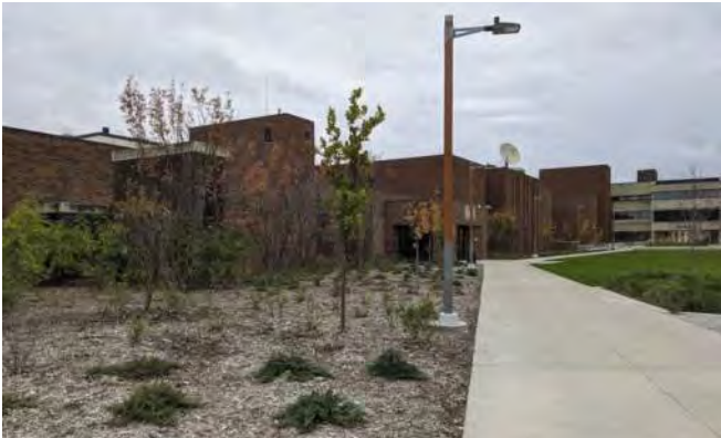
Wood Light Poles in South Courtyard
