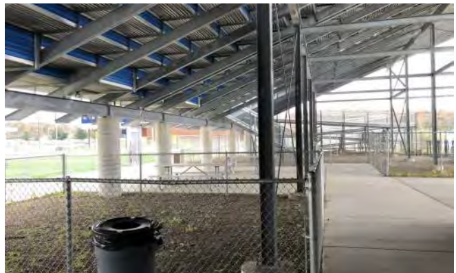
Area under Bleachers, outside of the Support Building
