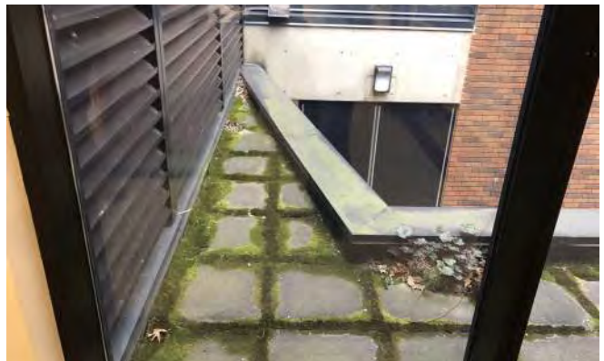
Roof visible from building corridor
