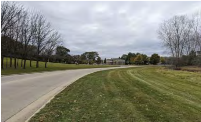
Pedestrian Connection Missing Along College Parkway
