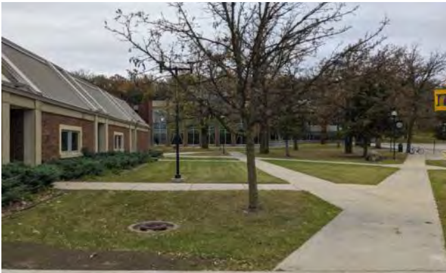
West Side of Main Campus Building
