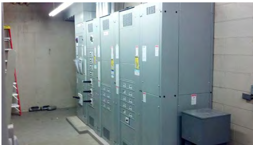
Typical Building Switchboard Figure 3-3
