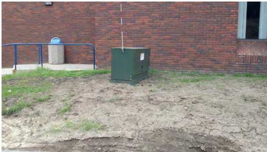
Typical RPU Junction Cabinet Figure 3-1
