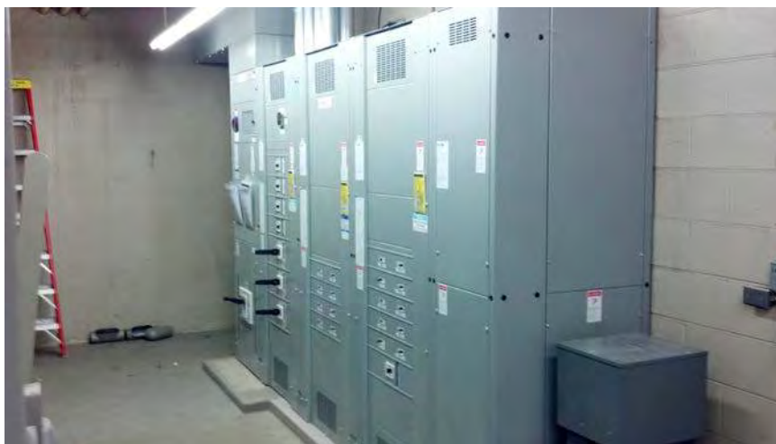
Typical Building Switchboard Figure 3-3
