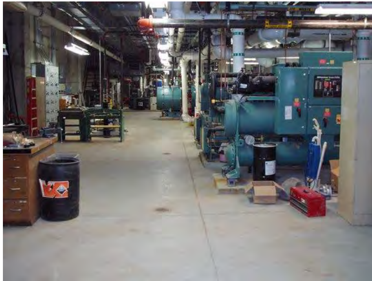
Existing Chillers in Mechanical Room ST006 Figure A-3
